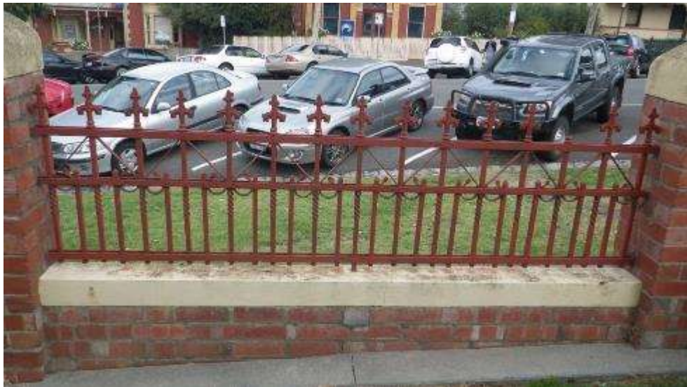
Figure 32 The wrought iron fence with cast iron spear points.
