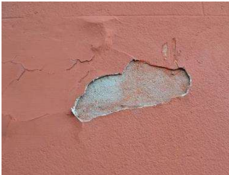
Figure 80 Paint lifting from render on the north wall of the Master's Residence
