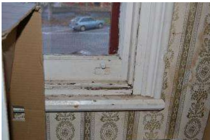
Figure 89 Damage from falling damp in the small tower room.
