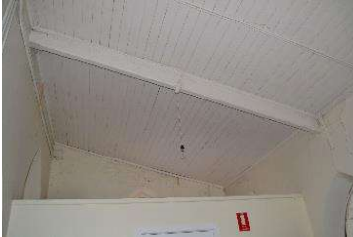
Figure 126 Lining board ceiling of the Vestry
