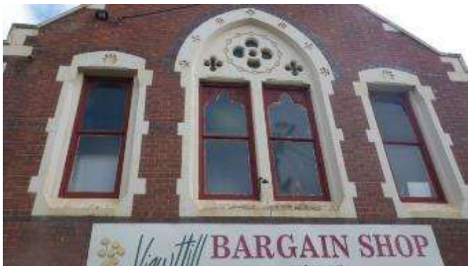
Figure 99 Decorative plate tracery on the front window.
