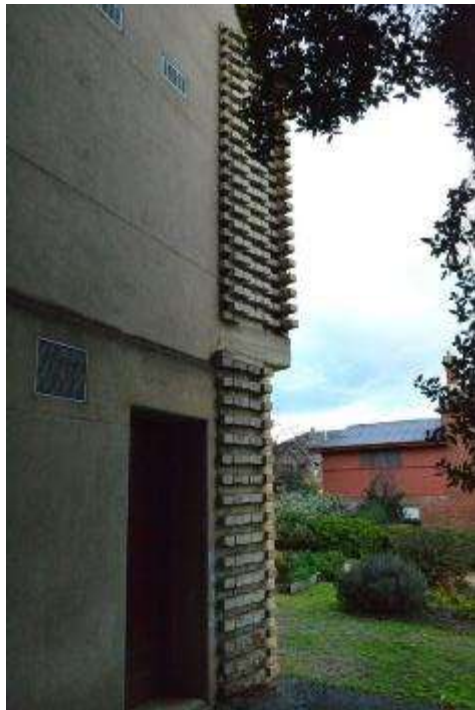
Figure 140 Temporary end wall ready for curved chancel end to be keyed in.
