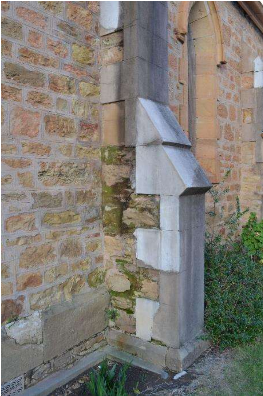
Figure 135 Falling damp from rusted out gutters is causing deterioration in the stone.
