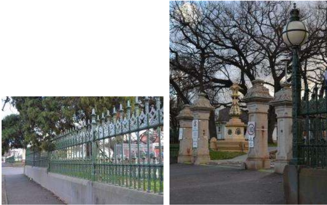
Figure 31 Bendigo Hospital fence, typical scroll pattern backstay can be seen behind it.
