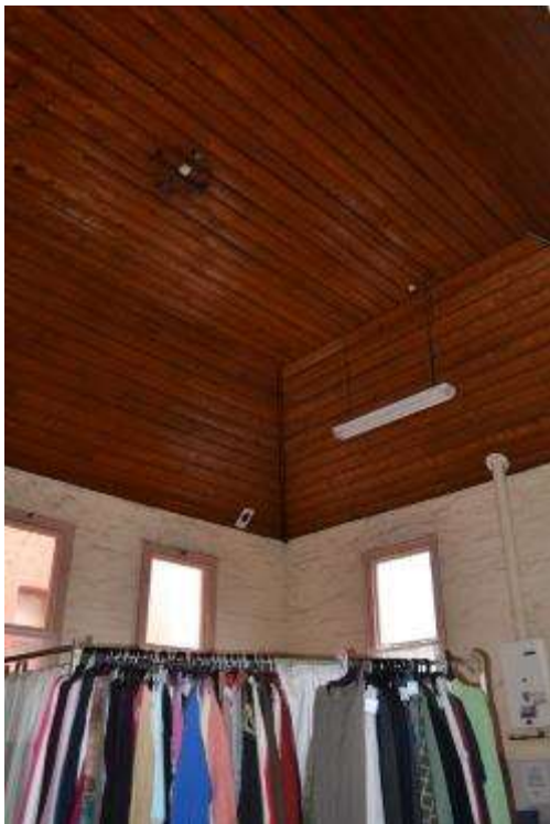
Figure 110 Coved ceiling of varnished lining boards in the back classroom.
