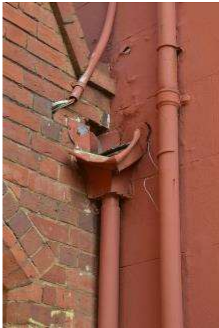
Figure 82 Blocked box gutters and downpipes, broken rain head and delaminating render
