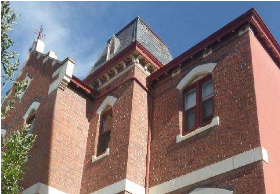
Figure 77 Mansard roof, front wall and finial, Master's Residence
