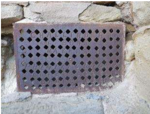
Figure 71 (Left) Air brick in All Saint's church wall by Challinder's Phoenix Foundry Bendigo
