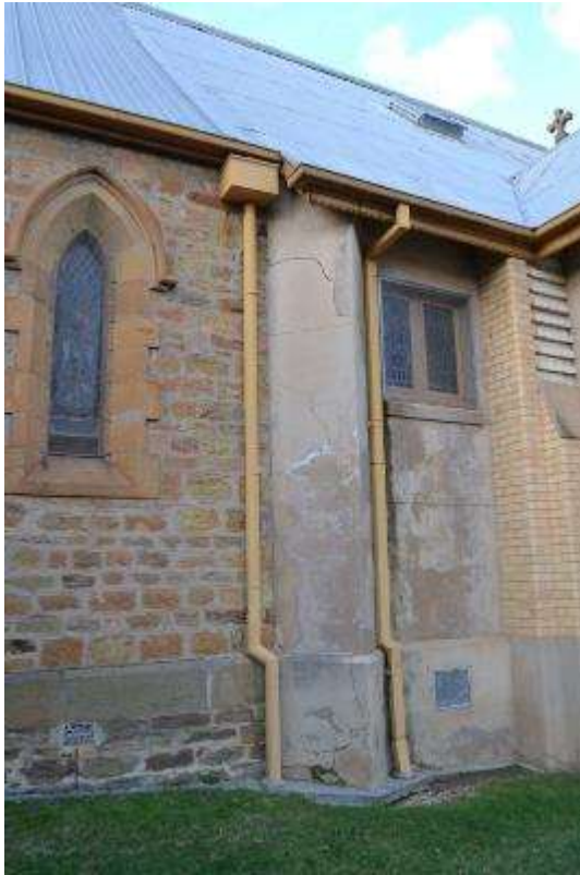
Figure 139 The junction of stone and brick on the southern side of the church.
