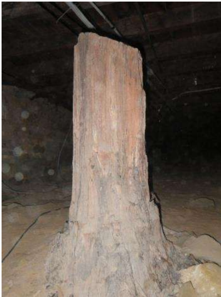
Figure 119 Ironbark stump under the church.
