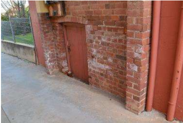
Figure 81 Salt damp causing fretting of mortar and bricks under the Gothic archway.
