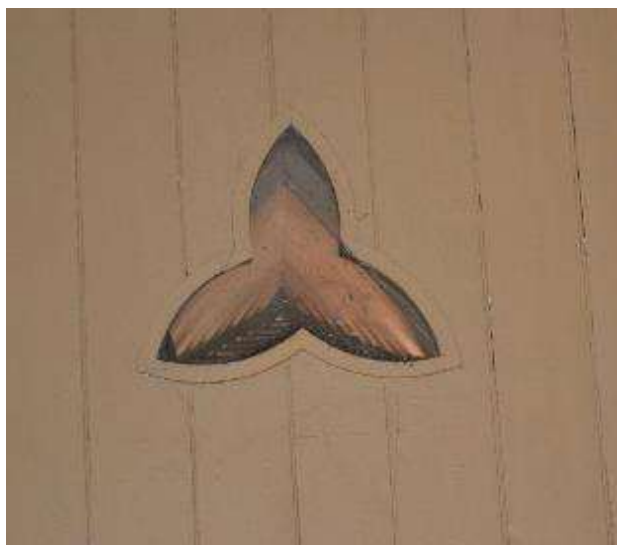
Figure 122 Roof vent in the chancel.
