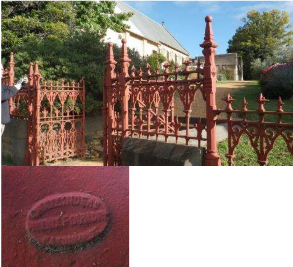
Figure 72 (Top) W C Vahland designed fence with Malmsbury stone plinth, cast at Challinders Phoenix Foundry. Challinders Phoenix Foundry mark (below)
