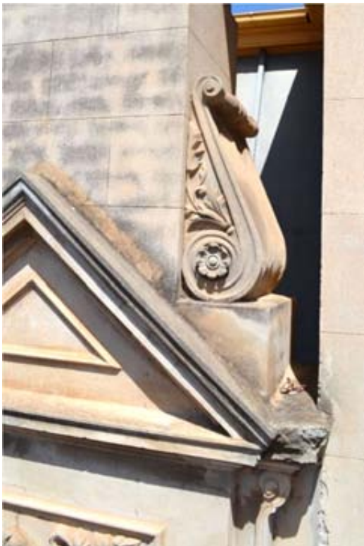
Figure 73: Remnant lime wash, Chimney on the walkway, First Floor.
