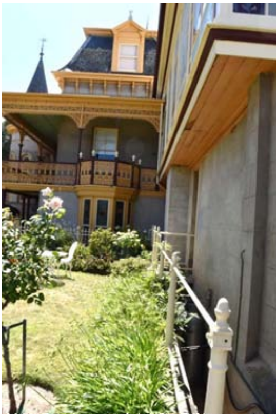
Figure 88: Conservatory cantilevers over former kitchen walls
