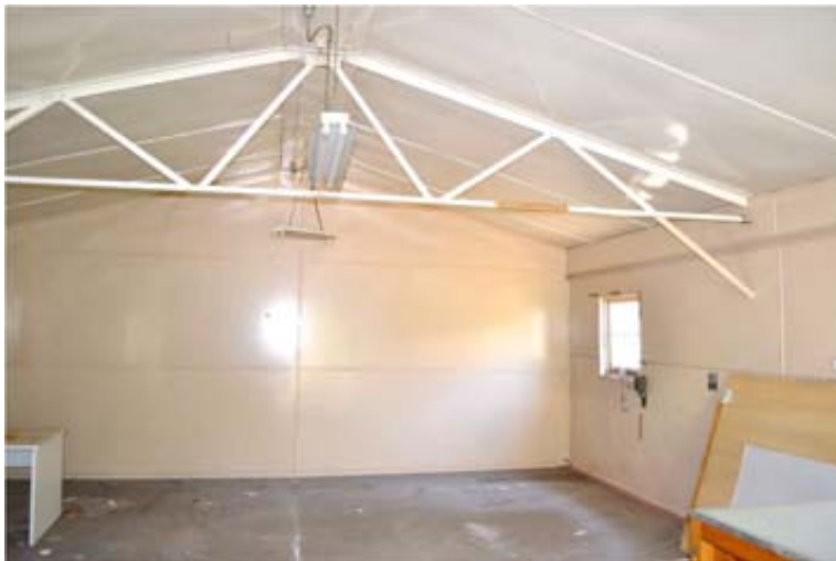
Figure 271: Steel truss inside the P1 hut
