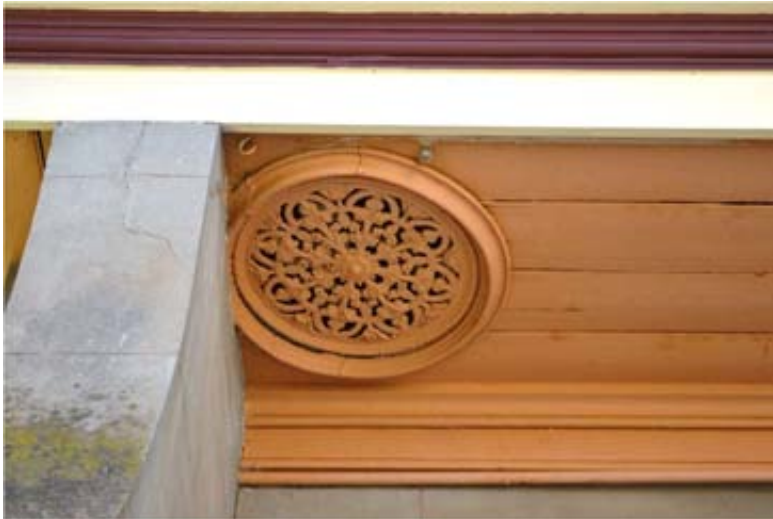
Figure 87: Original cast iron vent and soffit on West side of Conservatory.
