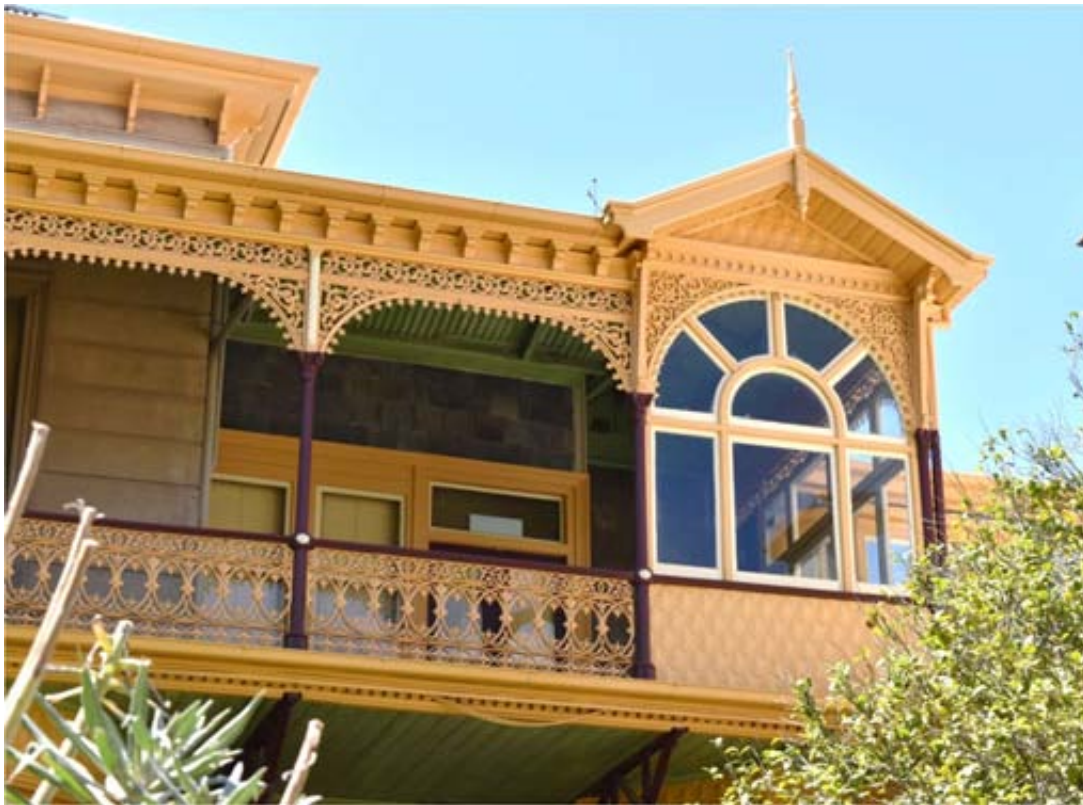
Figure 83: Queen Anne style timber gables and fish-scale pressed metal balustrading
