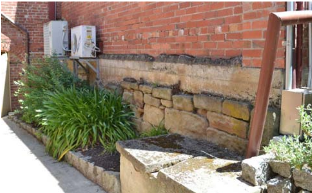
Figure 279: Stone foundation of Ballerstedts' crushing battery
