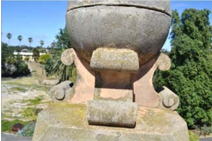
Figure 72: Remnant biscuit coloured lime wash on Roof Deck ornament.
